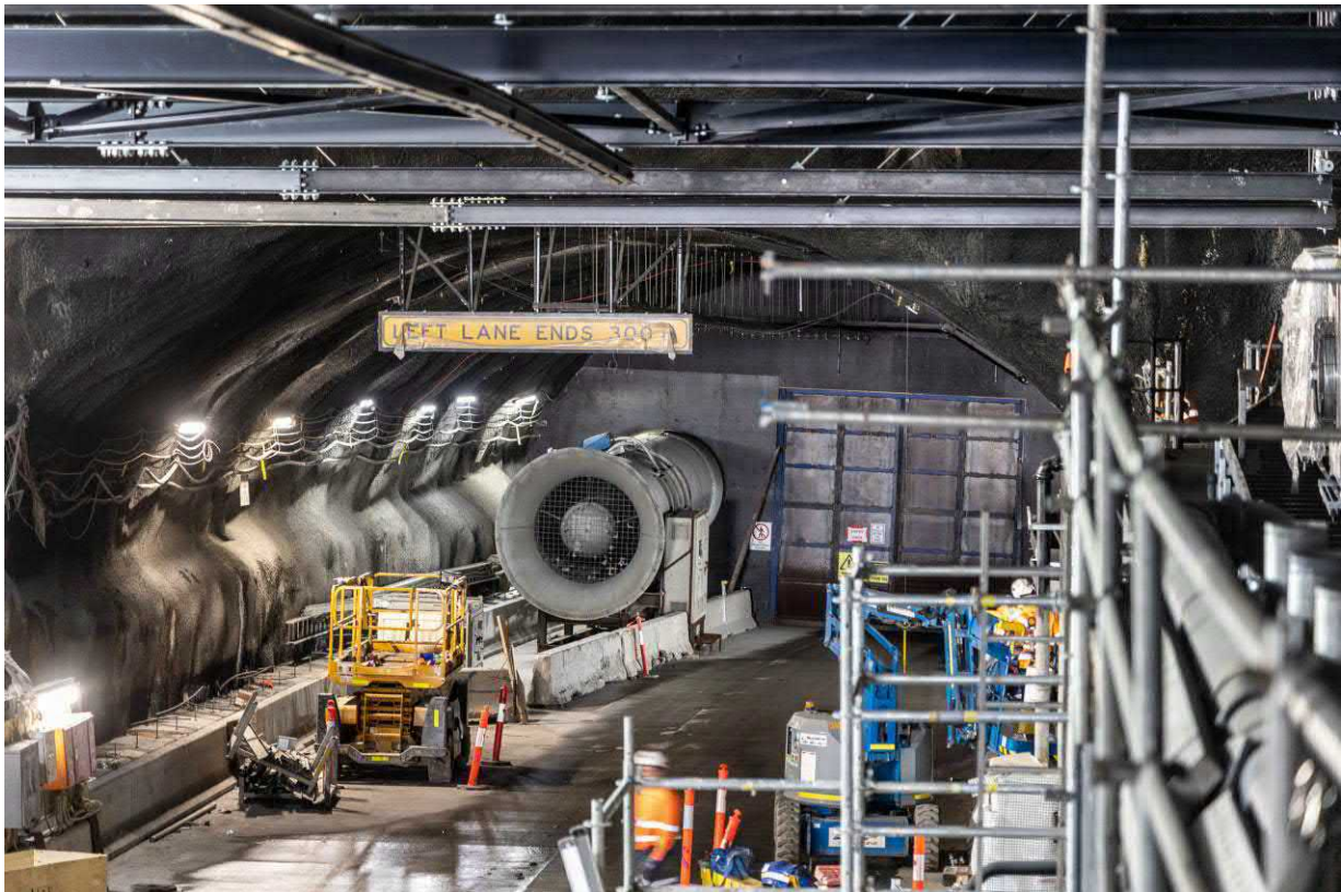
Figure 2-2 – M&E works underway at Haberfield, May 2022.
