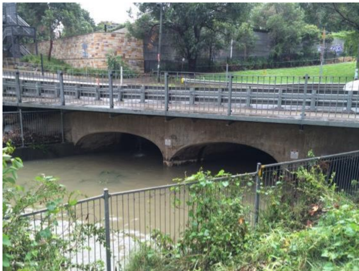
Plate 11 Culvert and footway from southern bank
