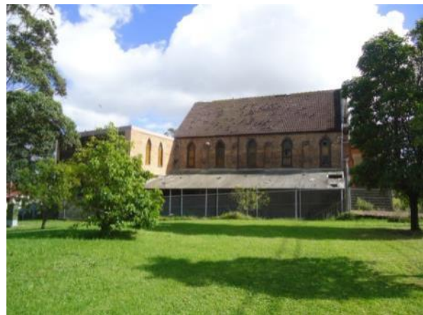
Plate 49 St Mary/St Mina Coptic Orthodox Church showing rear addition. View north.
