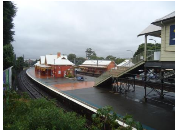
Plate 14 Arnccliffe Railway Station from footbridge
