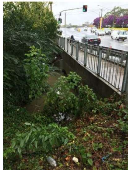
Plate 12 Downstream side of culvert from northern bank
