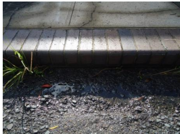
Plate 46 Example of Brick guttering in George Street.
