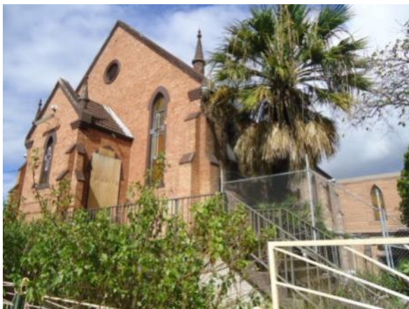
Plate 48 St Mary/St Mina Coptic Orthodox Church. View of front façade. View south west.
