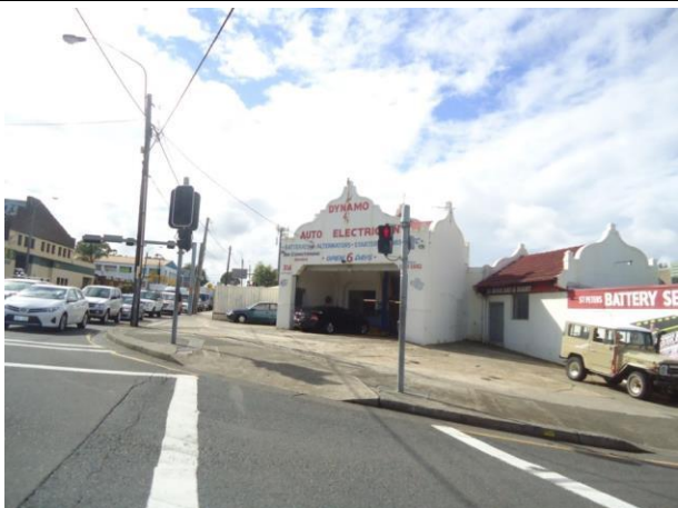
Plate 71 Service Garage (Dynamo Auto Electrician) View north east
