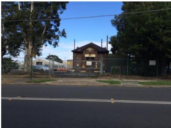
Plate 54 Huntley Street Sewage Pumping Station.
