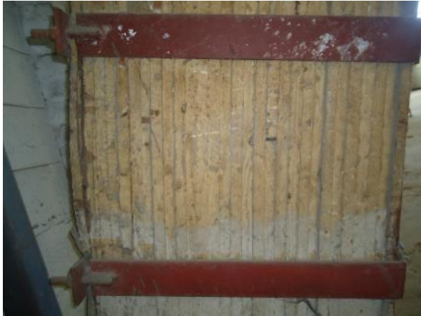
Plate 85 Detail of the laminated timber supports held together with 'D' bolts.
