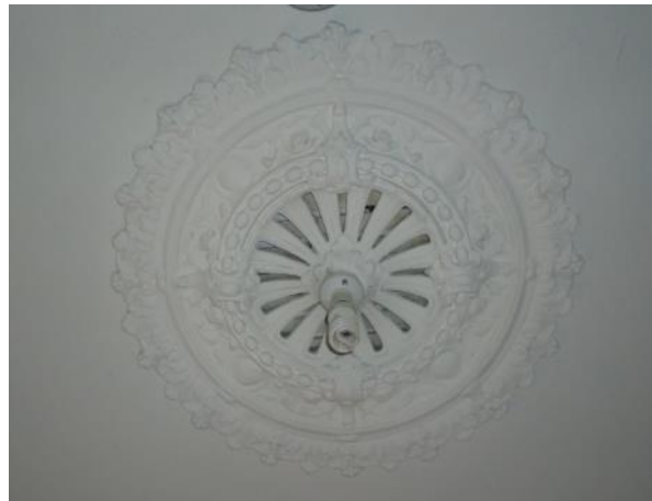
Plate 65 Interior of 44 Campbell Street. Ceiling rose in living room with lathe batons behind
