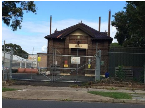
Plate 55 Huntley Street Sewage Pumping Station.
