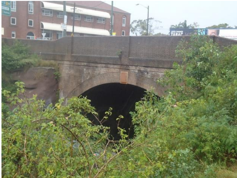
Plate 21 View of Forest Road Overbridge from Wardell Street looking north
