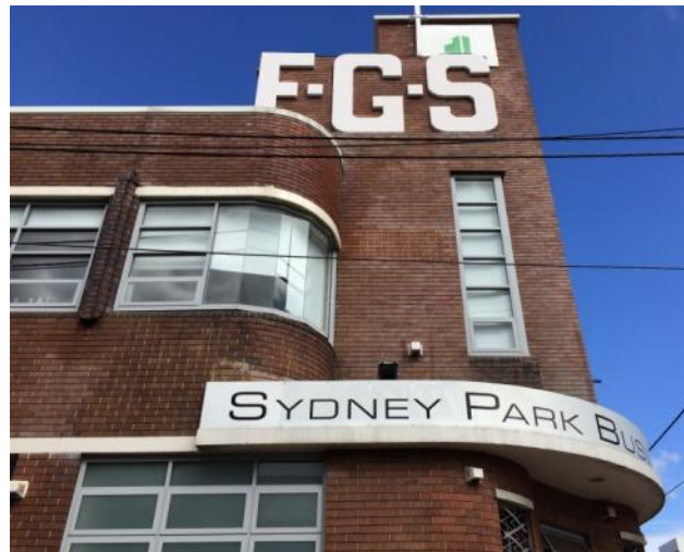
Plate 53 Detail of the Frank G Spurway Building from Maddox Street.
