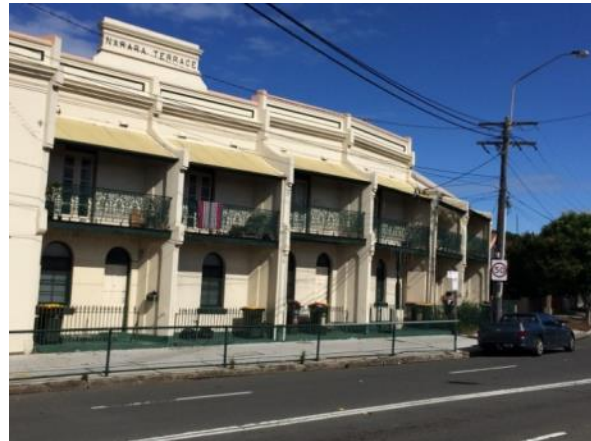
Plate 70 Detail of Narara Terrace, No. 8-18 Unwins Bridge Road.
