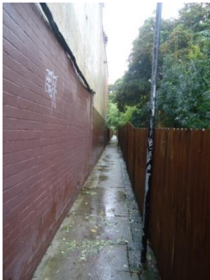
Plate 25 Glenevie Lane looking north west towards Barden Lane
