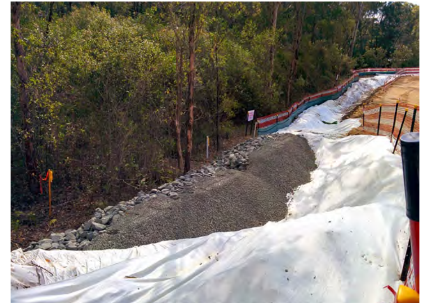
PHOTO 1: ROCK FILTER DAM EXAMPLE
