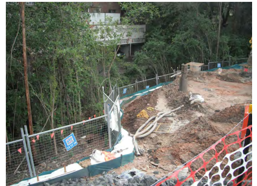
PHOTO 2: MODULAR SEDIMENT TRAP EXAMPLE
