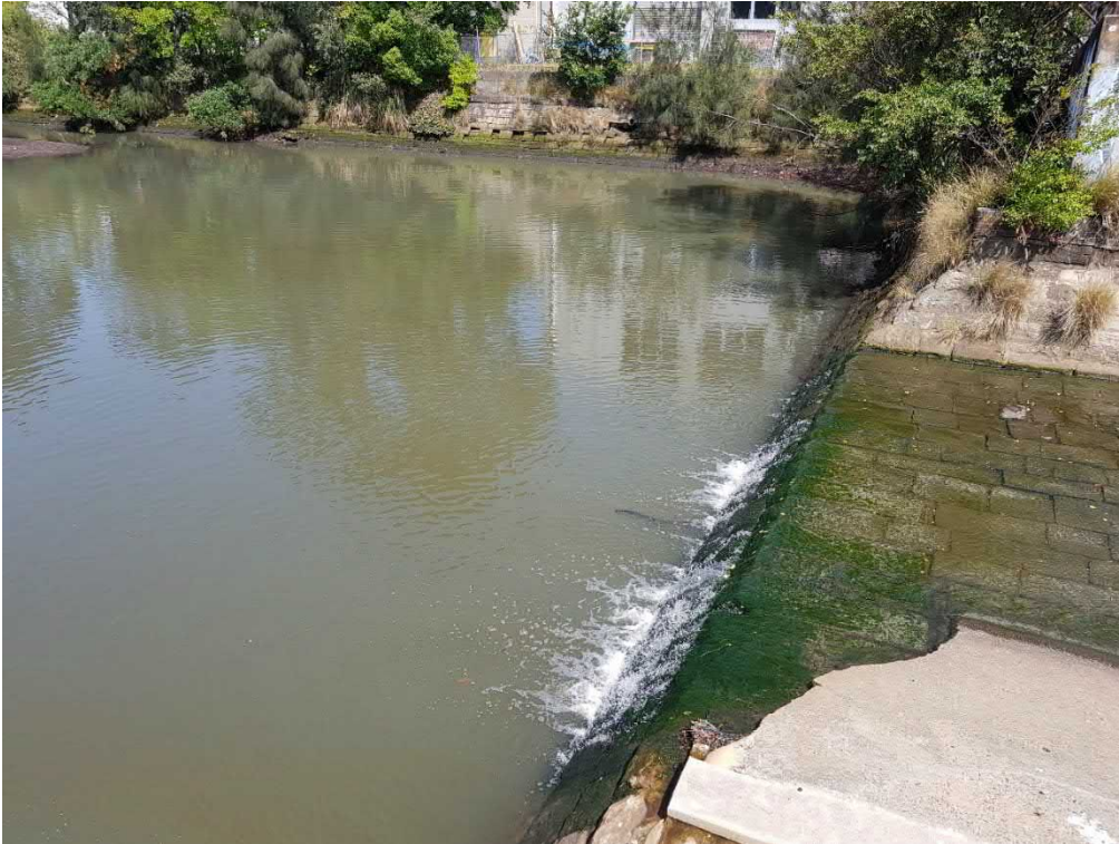
Photograph 5.6 Weir between Sheas Creek (control site) and Alexandra Canal
