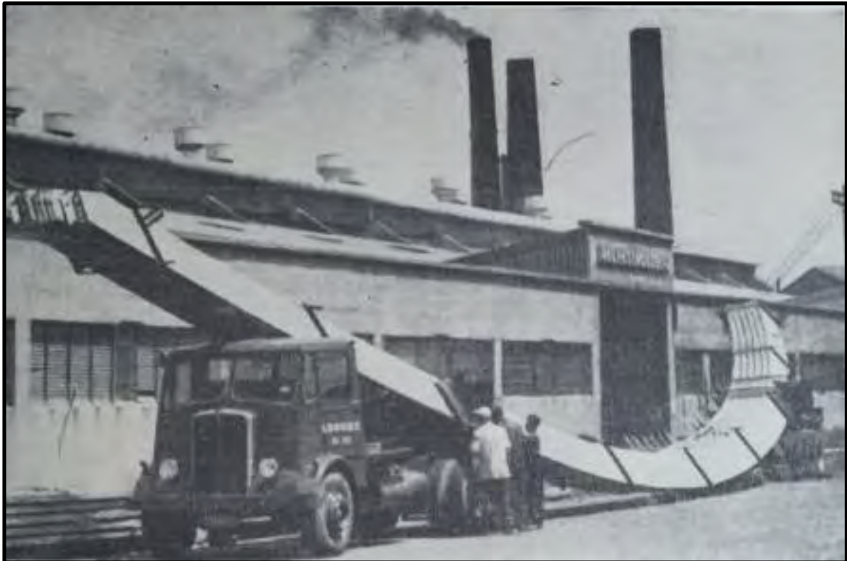
Figure 21. Laminated timber arches manufactured by Ralph Symonds Ltd, Sydney, for transportation to Melbourne for the Neon Industries building. (Source: "120ft Laminated Timber Arches, Transported from Sydney to Melbourne. Building Lighting Engineering, 24 March 1955 p.33. NSW State Library).
