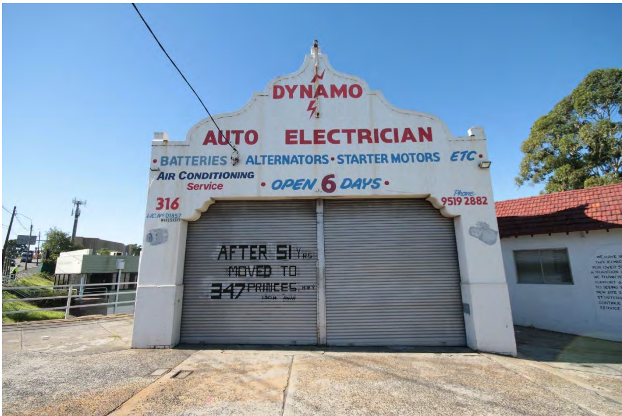
Figure 4. Condition of the Building façade in 2016.
