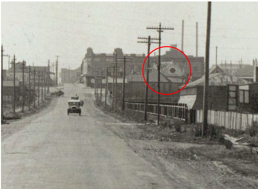
Figure 10. Canal Street, St Peters, c.1934, showing a southern parapet on Canal Street, outlined in red (source: State Archives and Records New South Wales, call number FL 124060).
