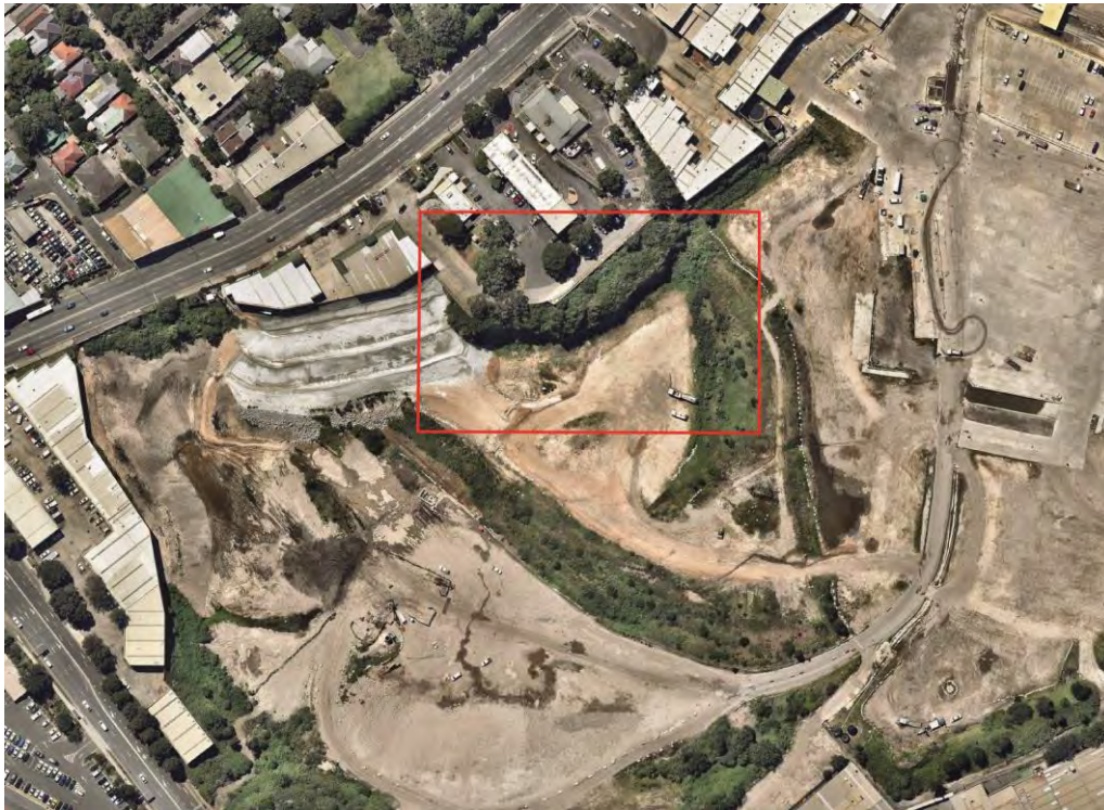
Figure 2. Aerial view with subject property outlined in red (Source: NearMaps accessed 12.08.16).
