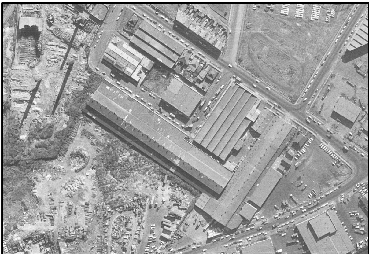
Figure 13. Aerial photograph, 1970. Shows full building as per early 1950s planned layout. (Source: NSW Department of Lands).
