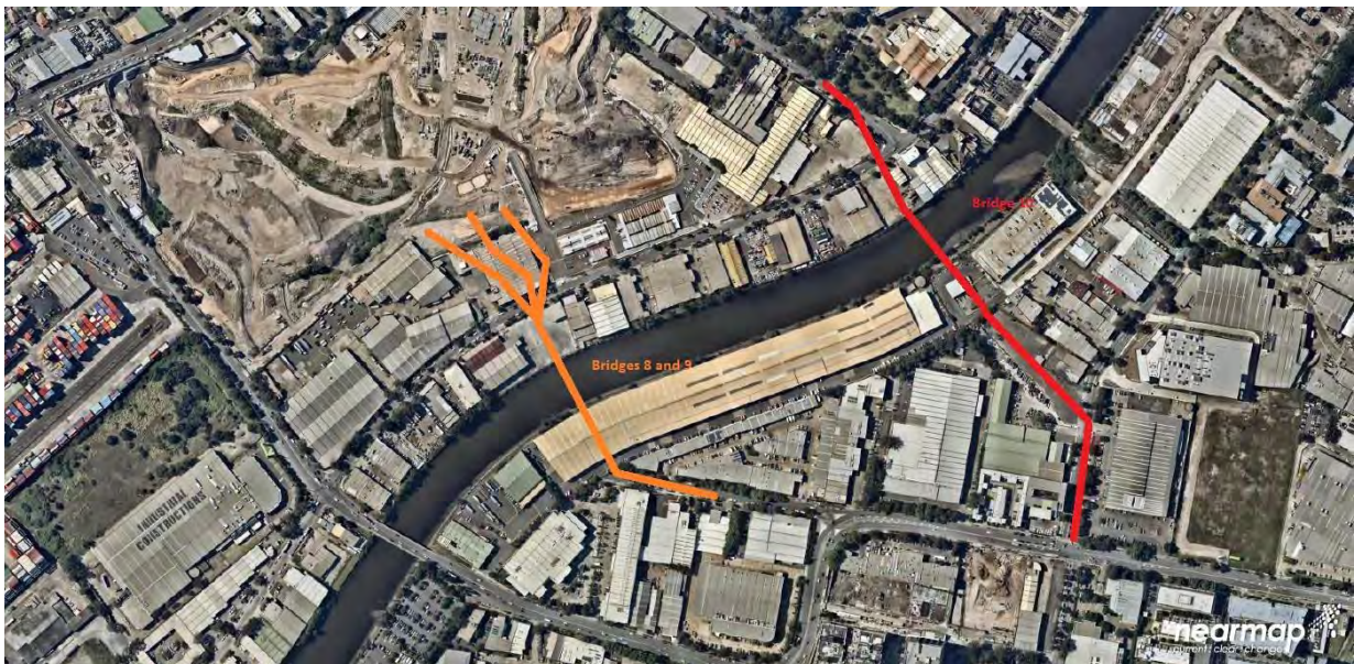
Figure 3: Aerial view of Bridges 8 & 9 (outlined in orange) and Bridge 10 (outlined in red) (Source: NearMaps, 2017).
