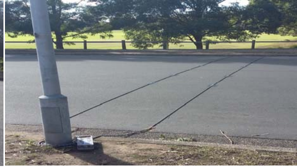
Figure 5: Close up picture in Wirega Avenue
